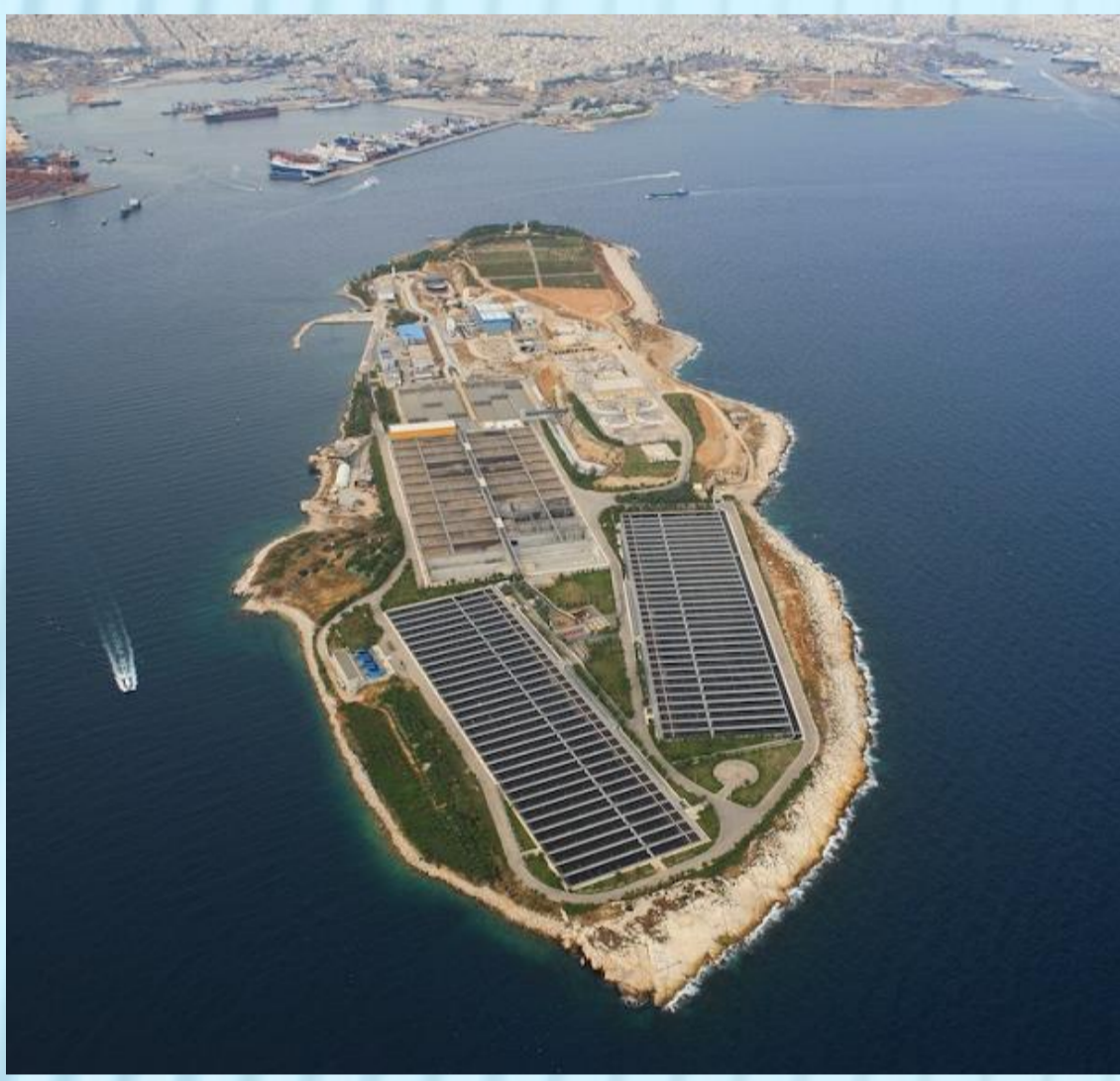
Figure 2: Psytalia wastewater treatment plant
