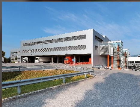
Plant 4 in Bregenz
