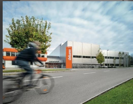
Plant 6 in Gaissau
