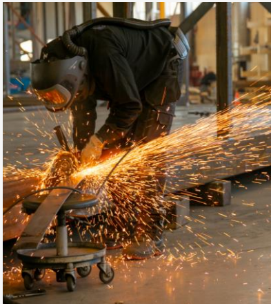
1. Steel frame manufactured in welding shop
