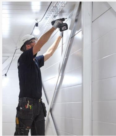
3. Walls, floors, panels mounted
