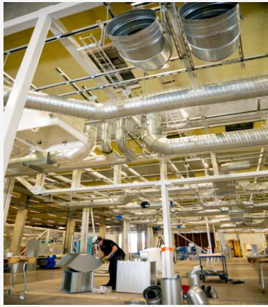
2. Installations of HVAC, electricity, piping etc
