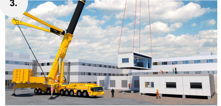
Placement of the modules
