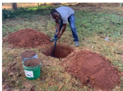
b. Separate top and bottom soils
