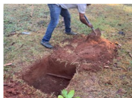
f. Start re-filling the hole with the mixture
