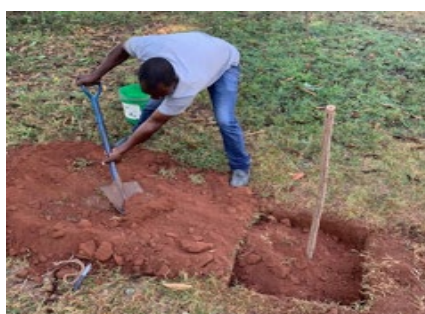
g. Complete re-filling the hole with bottom soil and insert a peg to mark the center of the dug hole
