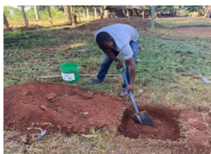
g. Complete re-filling the hole with bottom soil and insert a peg to mark the center of the dug hole
