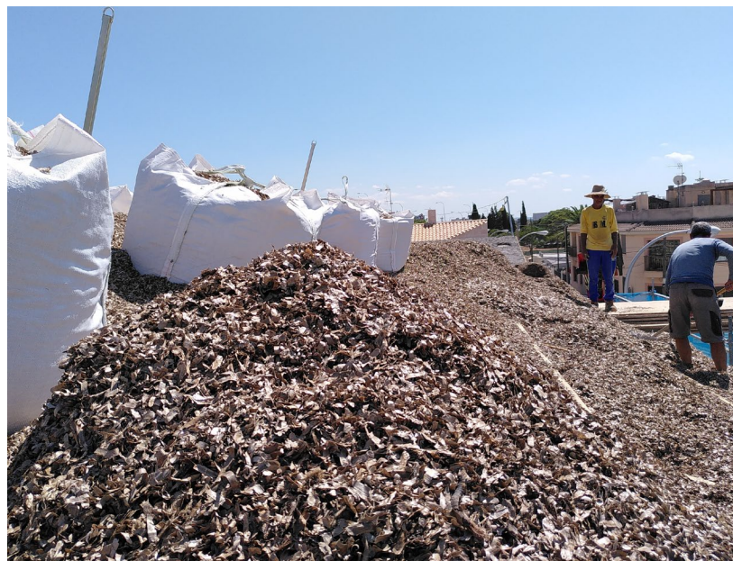
Posidonia insulation at 167 dwellings
